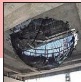
Fall Protection & Debris Nets
