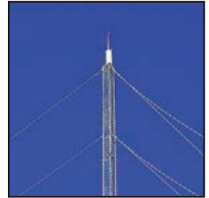
Antenna Guy Lines
